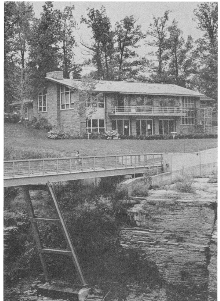
Noyes Lodge, at Triphammer Falls, gets post-fire repairs.
