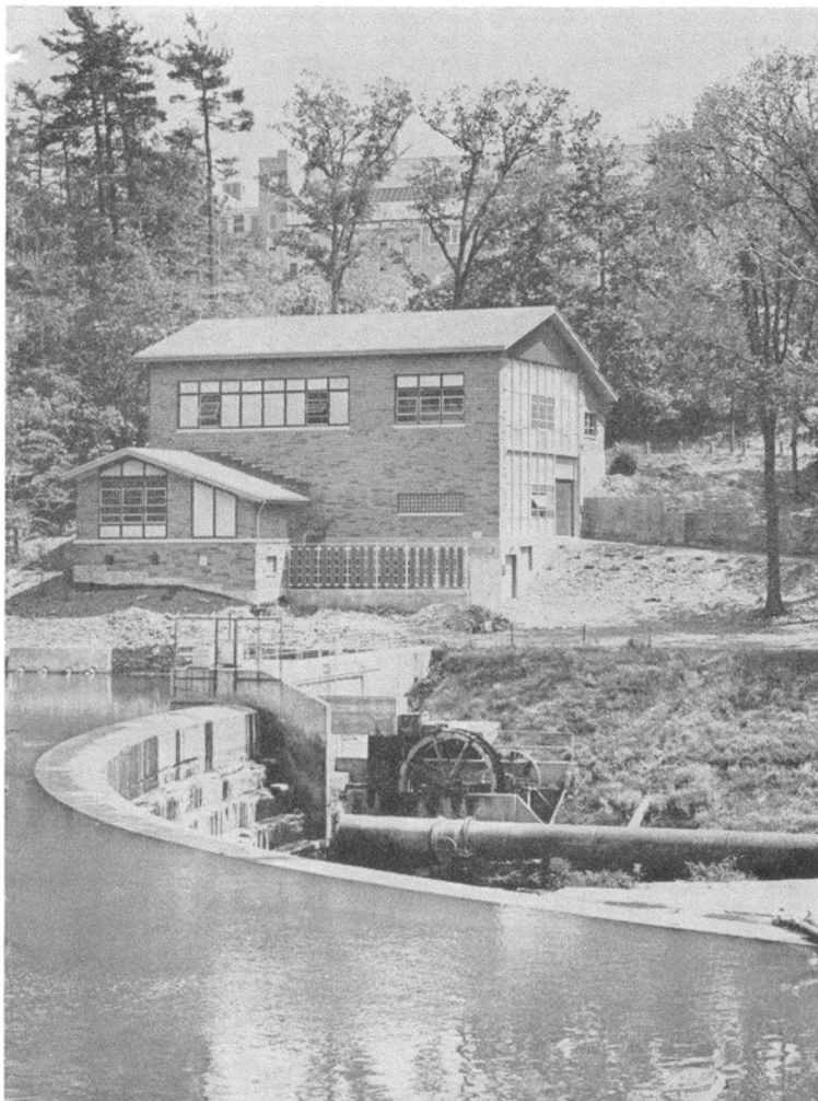
Chilled Water Plant is a new fixture on the south shore of Beebe Lake. July 1964
