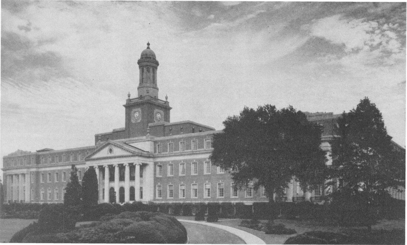
Massachusetts Mutual Home Office
