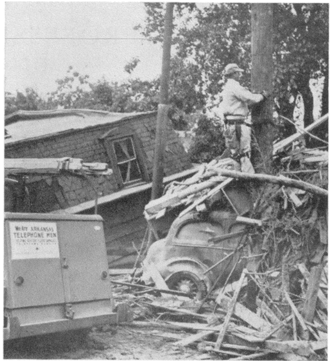
Meeting the Emergency. Telephone people not only worked valiantly to restore service but to keep it going. Dikes were thrown around telephone offices. Switchboards raised above rising waters. Emergency power plants set up. Mobile radio telephones rushed to towns where telephone offices were washed out.
