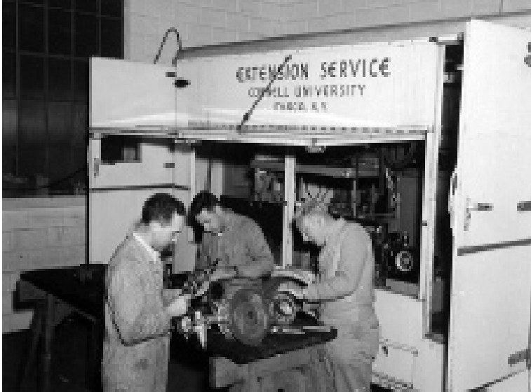
E. Stanley Shepardson, Extension instructor, left, with district agricultural engineers Hollis R. Davis, center, and William F. Millier, repair electric motors in the Chemung County Highway Garage in Big Flats after a flood on May 28, 1946.
