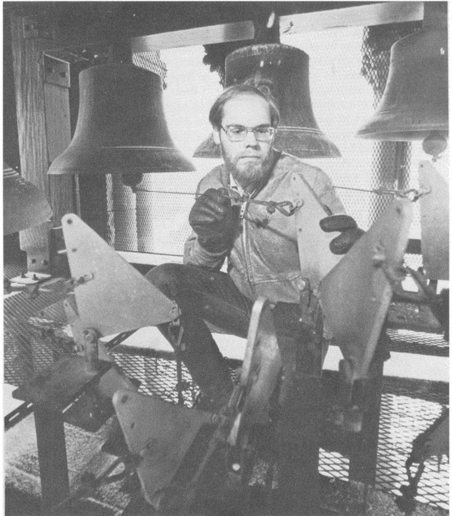
hour and changing of classes. But more urgent jobs have been undertaken: installing new steel beams to support the weight of the bells, a new playing console that is nearly complete, screens around the belfry, renovation of the room and a new floor, a fire alarm, new wiring, and the repointing of masonry on the outside of the tower. Much of the money has come from the university's buildings and properties budget, some from a memorial endowment set up in the late 1930s.
