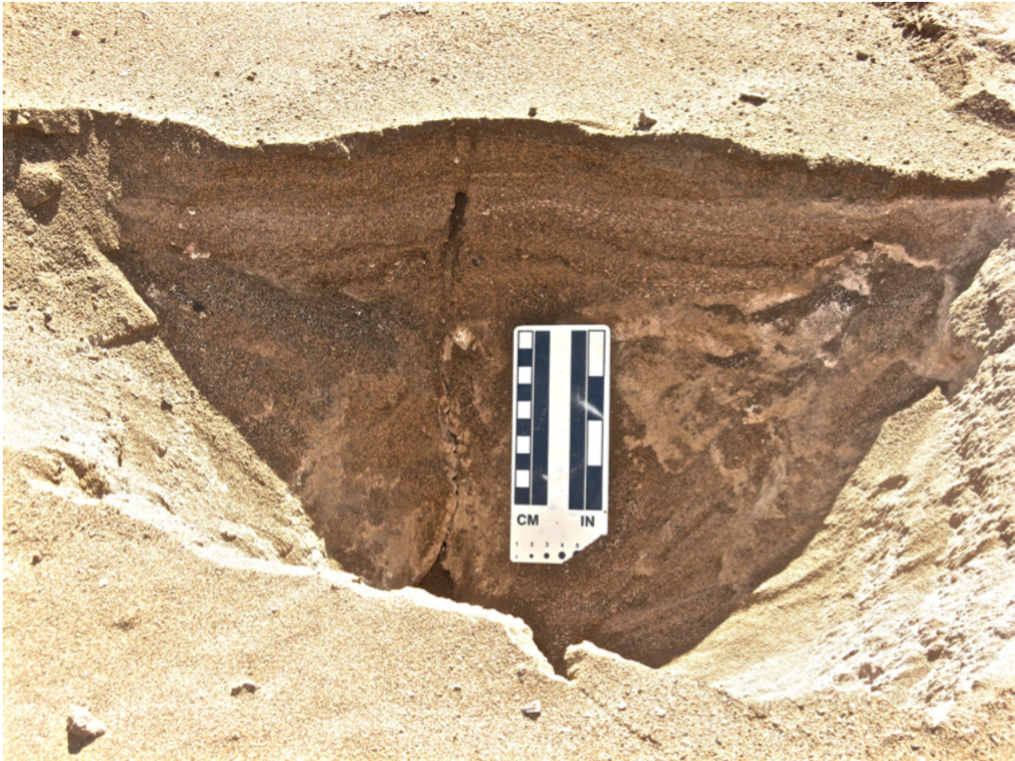
Figure C.8: Excavated crack profile showing that walls degrade near the surface. This photo is of a crack opening produced during the 2007 Mw 7.7 Tocopilla earthquake. Crack opening in the more competent material at the depth of the scale may better reflect the coseismic strain than the apparent crack opening in the looser sand. Loose eolian sand accumulated in an old surface crack depression has enhanced the new crack opening, which overlies a very fine crack in gypsum fill (lighter material where the scale is located).
