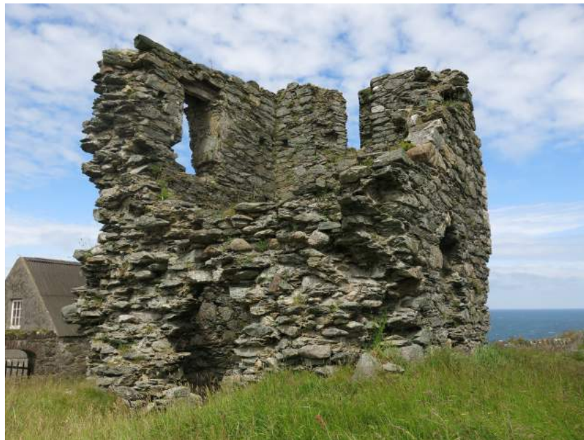
Figure 12: Ruins of St. Mary's Abbey Tower, Bardsey Island
