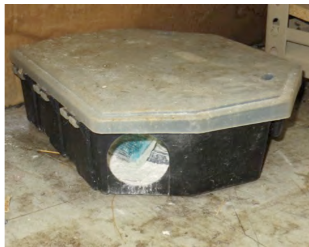
Figure 2. Excessive use of tracking powder in bait station, with a 0.5 cm layer of material. An additional violation is the failure to secure the soft bait rodenticide in the station.
