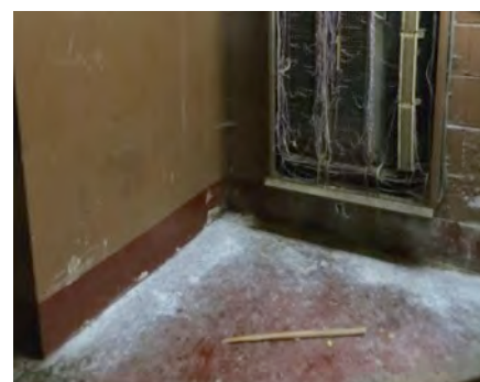
Figure 3. Egregious violation of label, exceeding location placement, amount of product, and patch size specifications.
