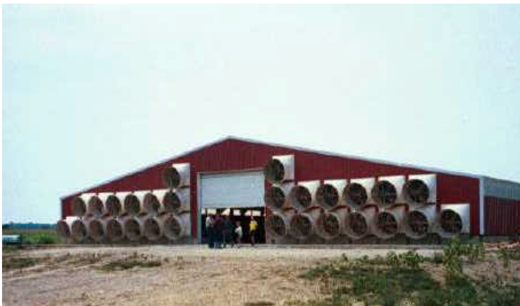
Figure 2. Large tunnel fans on a six-row freestall barn.
