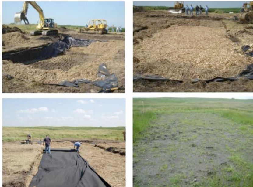
Figure 3. The images above are various depictions of a woodchip denitrifying bioreactor from the initial development stage (top left) to the finished project in the bottom right corner (South Dakota Corn, 2013).
