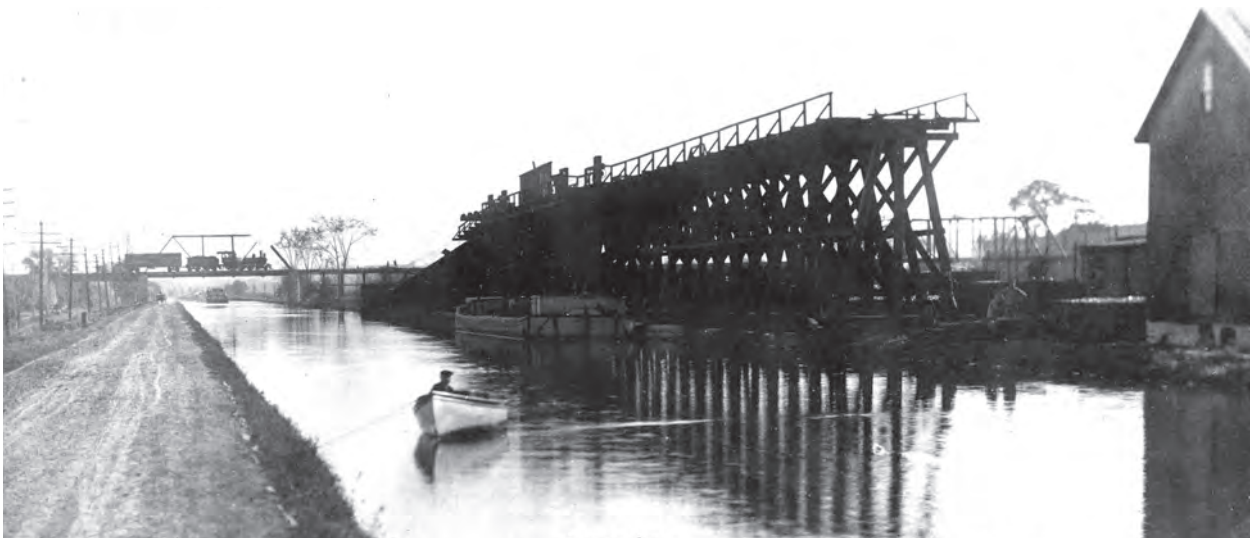
Elmira, Cortland & Northern coal trestle built in 1885 and 1886 for unloading coal into Erie Canal barges, a breakthrough that greatly increased freight tonnage for the line.
