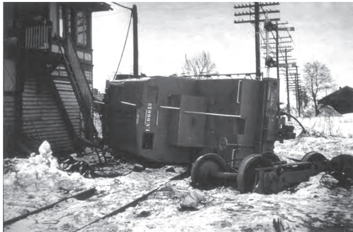
Snowplow rests near steps of the New York Central tower in Canastota after a runaway trip downgrade from near Perryville in 1958.
