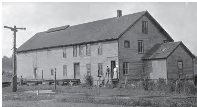
Sheds Corners Station looking west, located just south of the 1,390-foot summit of the EC&N between Cortland and Cazenovia.
