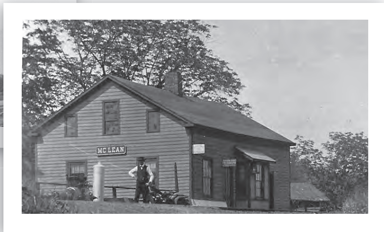
BELOW: McLean station with building on west side of track; main track in the direction of Cortland.
