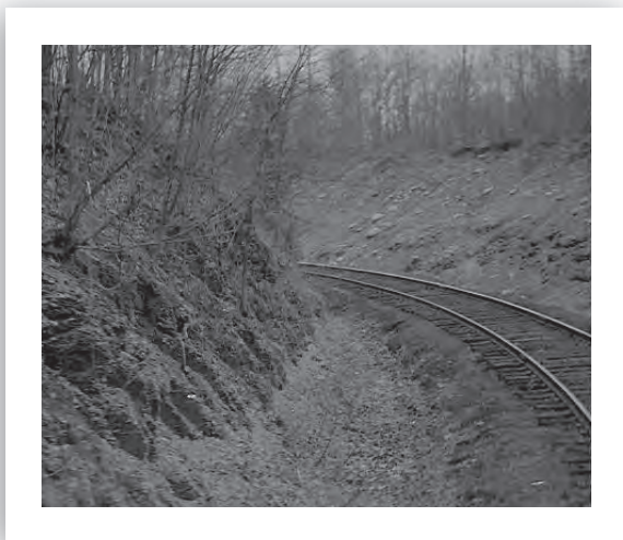
Fireman's view of the 15 m.p.h., 15-degree curves on the steep grade south of Canastota.
