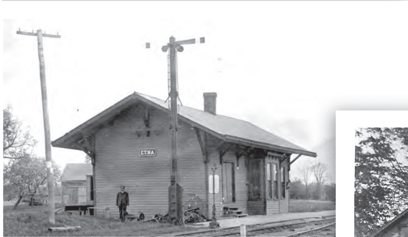
LEFT: Etna station with the main track to the right in the direction of Freeville.
