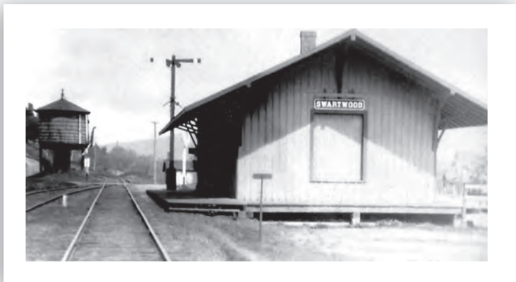
Swartwood Station looking upgrade toward Park Station
