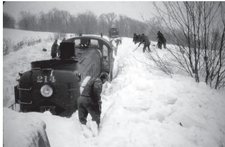
Engine 214 with snowplow ahead is buried in a snow-filled cut headed north on a grade known as Falls Hill between Chittenango Falls and Blakeslee. The Cortland yard Engine 115 in the distance waits for snow-shovelers to clear snow from around the locomotive.
