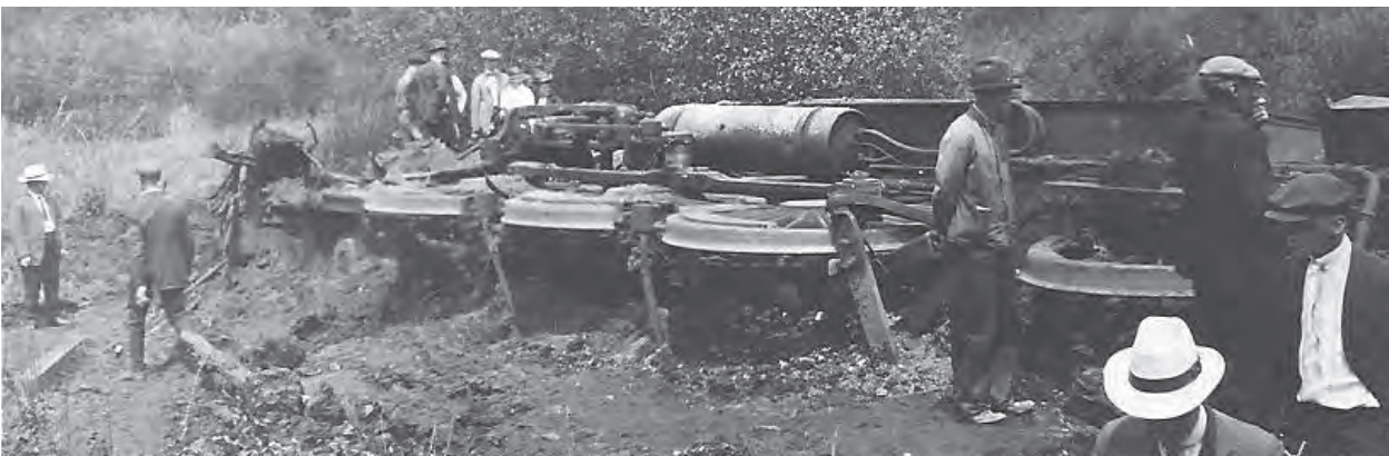
Bystanders and railroad personnel at the north end of the Van Etten yard after the May 1920 accident. Extra 1155 North with Engine 1162 assisting was traveling from left to right on the Swamp Siding when it derailed at the switch at the extreme right. Engine 2059 leading Passenger Train 6 traveled at 50 miles an hour from right to left and slammed into the tender of the freight train's lead Engine 1155 and into its second engine, 1162. From right to left are the fourth, third, second and first cars of Train 6 and two derailed hopper cars from Train 1155 North. BELOW: Train 6's Engine 2059 rests on its right side in the swampland, viewed from the Ithaca Branch main track.
