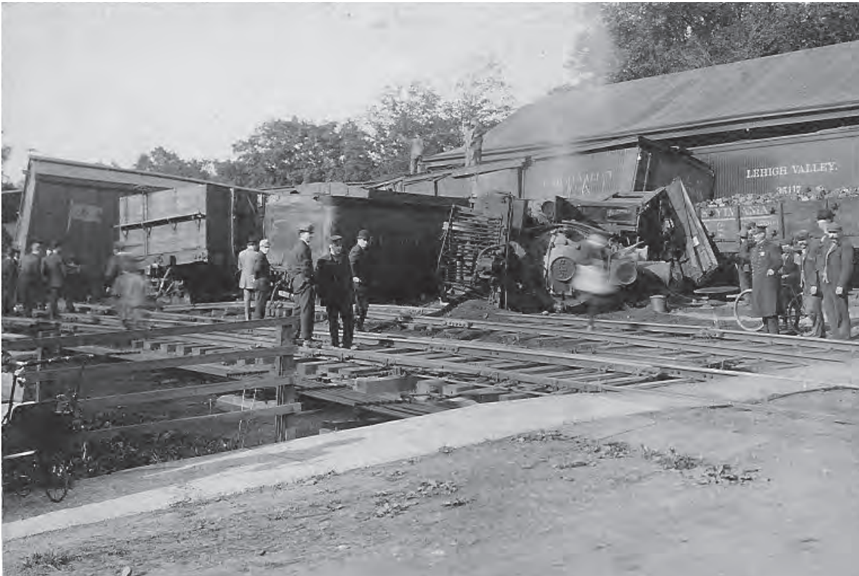
Results of a runaway train at Canastota on June 10, 1910, encountering a heavy derailer intended to keep LV trains from running across tracks of the West Shore RR.
