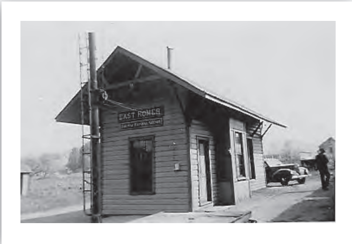
East Homer Station looking north.
