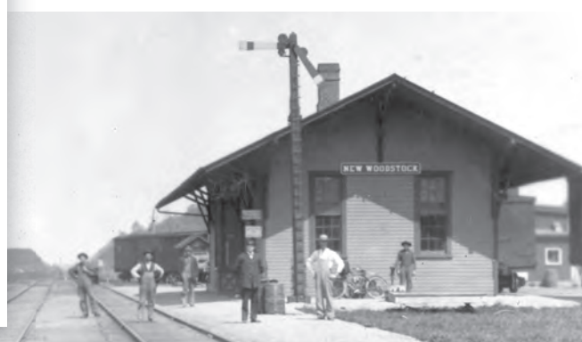
The station at New Woodstock looking north.
