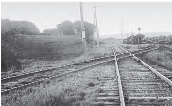
ABOVE: Caroline Junction, looking north with EC&N tracks crossing Delaware, Lackawanna & Western track from left to right. Signal tells which line's train has the right of way.
