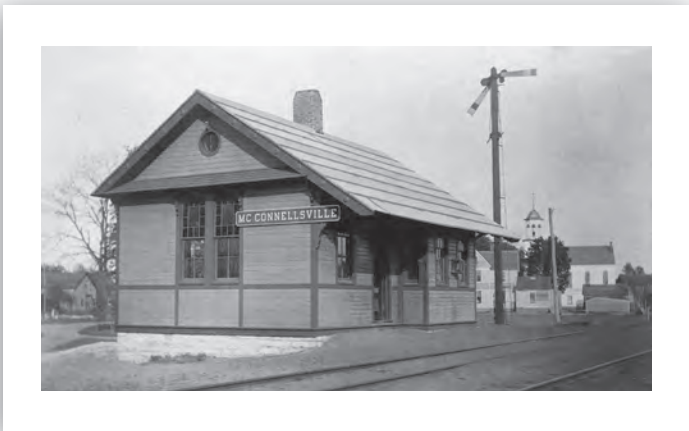
McConnellsville is one of the busiest stations on the Camden extension; the community is also served by the New York Central Railroad's Rome-Richland Branch.
