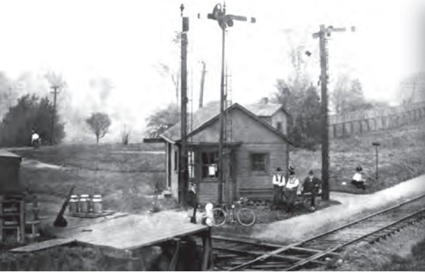
Rippleton Station with building in the northwest quadrant of the crossing. The Elmira and Cortland Branch track runs from lower left toward Cazenovia.
