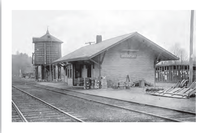
The Breesport station with track to the right in the direction of Erin.
